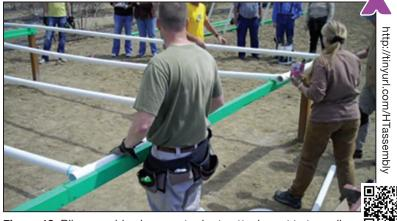
Figure 12. Rib assembly placement prior to attachment to top rail.
