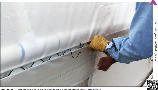
Figure 38. Holding the poly skin in the wiggle wire channel with wiggle wire.
