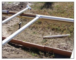
Figure 20. Scab over butt joint of base plate.
