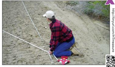
Figure 6. Checking the diagonal measurement of the structure.
