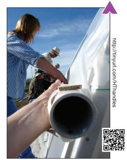
**Figure 39.** Attaching lath strips to rollup side handle.
