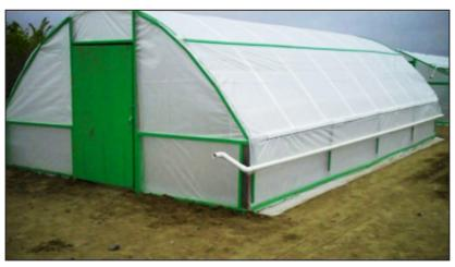
Figure 1. Completed 16' X 32' Hard-sided high tunnel.
