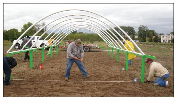
Figure 21. Establishing end wall layout.
