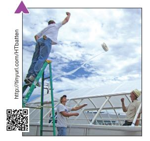
**Figure 40.** Throwing batten tape over structure for attachment between ribs.
