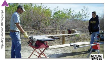
Figure 2. Ripping lath material.
