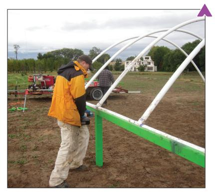
Figure 19. Removing the temorary side rail.
