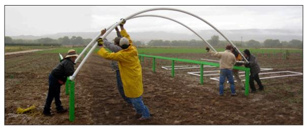
Figure 14. Method used to position rib assembly onto wooden base.
