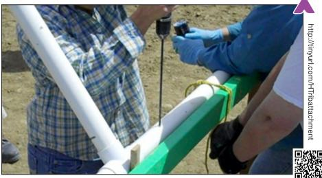
**Figure 15.** Attachment of Rib assembly to wooden base. Drilling hole for carriage bolt; note 3/8" lath spacer at joint and holding the rib in place with rope.
