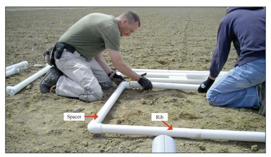
Figure 3. Spacer assembly first and adding the ribs.
